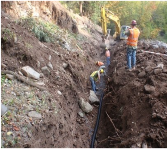
Drainage pipe placed before construction of the wall.
