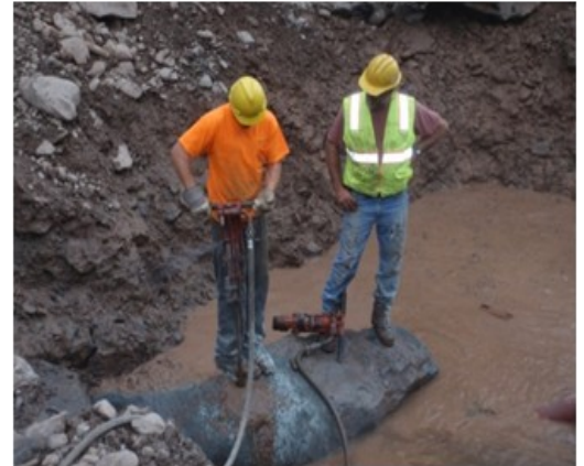
Rocks pinned to bedrock with steel rebar
